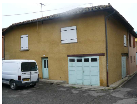
Maison centre village
